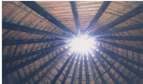
Interior of Ceiling
